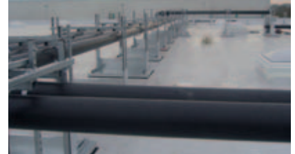
COOL-FIT ABS pipe installation on the distribution centre roof.
